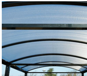
Robust roof framework with rainwater gutters
